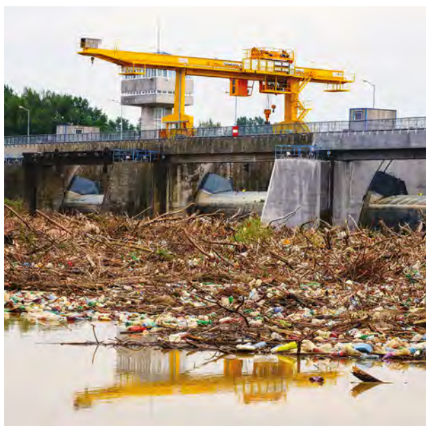
Plastic and driftwood accumulation after a flood in downstream Hungary, at the Kisköre hydropower plant (HPP). The temporary structure can be 3 meters thick and reach more than a hectare in overall size. Photo: Plastic Cup
